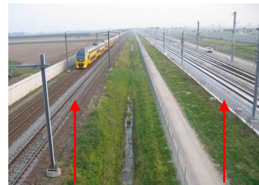
Figure 1: 1500 V DC track next to 25 kV AC track (HSL-Zuid)
