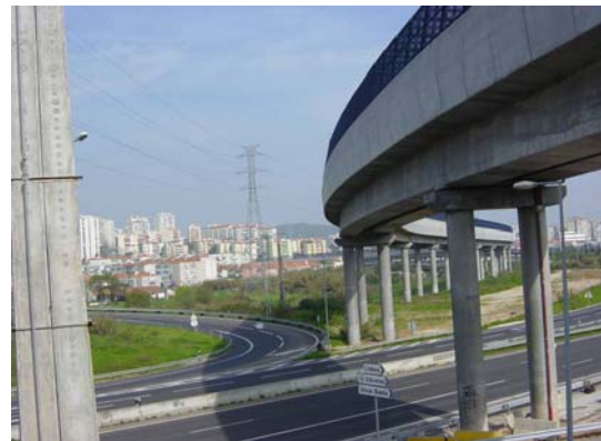
Fig. 2. HV Line in parallel and crossing metro viaduct
