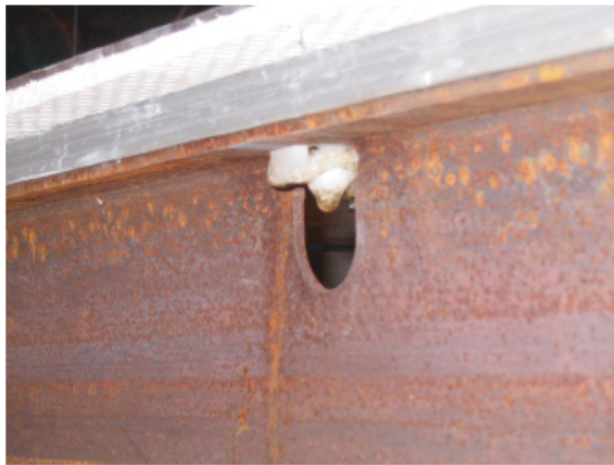
Fig. 9: The nylon bolt softens
