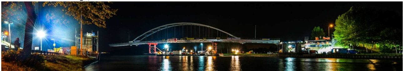
Figure 9. Installation during the night
