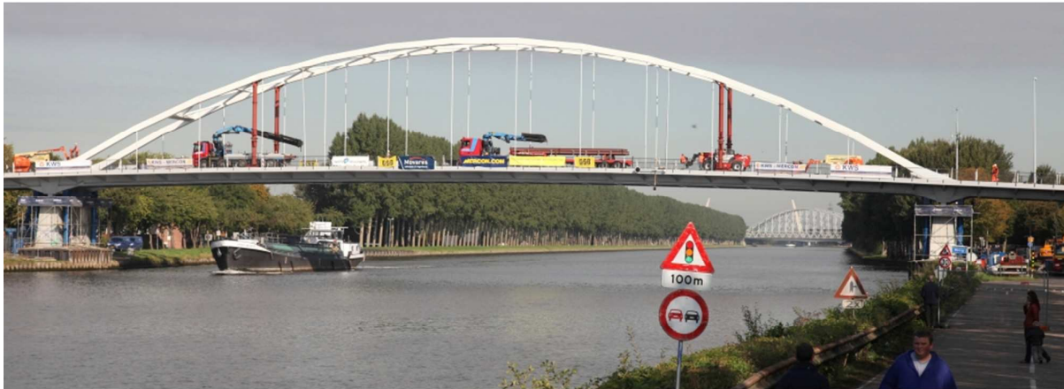
Figure 10. Removing temporary structures the day after
