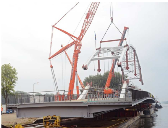
Figure 3. Assembly Arch to deck
