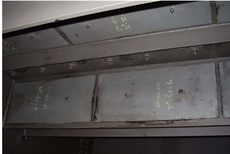
Fig. 4 Sandwich plates added to deck plate and stringer
