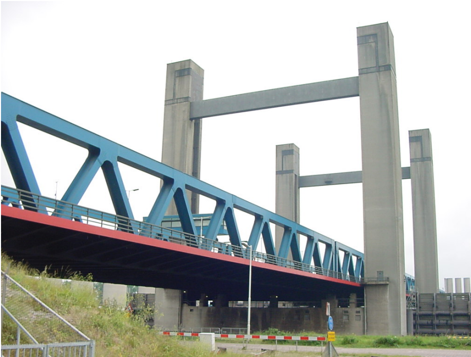
Fig. 11 Caland Bridge fit for service until the year 2020
