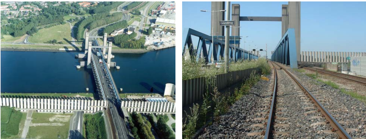
Fig. 2 Caland Bridge for rail and road, overview
