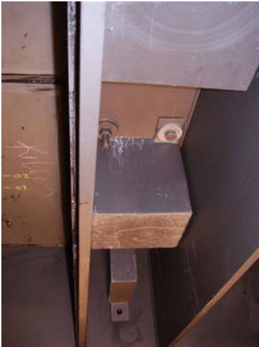
Fig. 3 Mass blocks under rail
