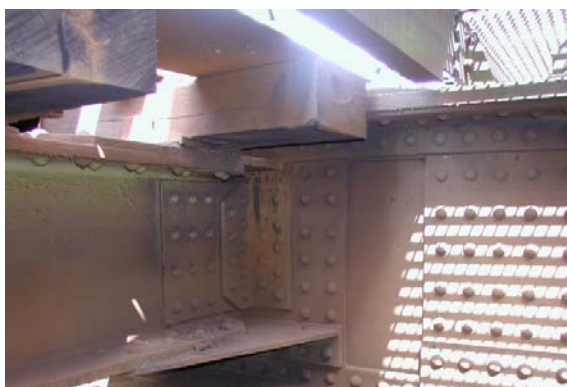
Figure 15. Traditional deck system
