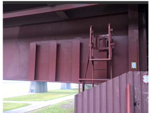
Figure 13. Strengthening of the web preventing local buckling, Kreekrak Bridge
