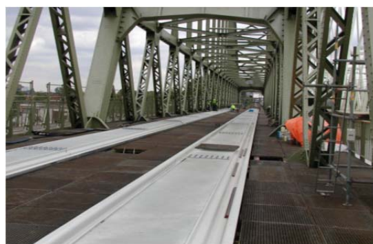
Figure 16. New silent bridge® decks
