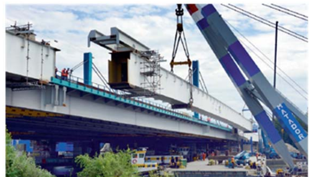
Figure 10. Installation of strengthening girder, Galecopper Bridge
