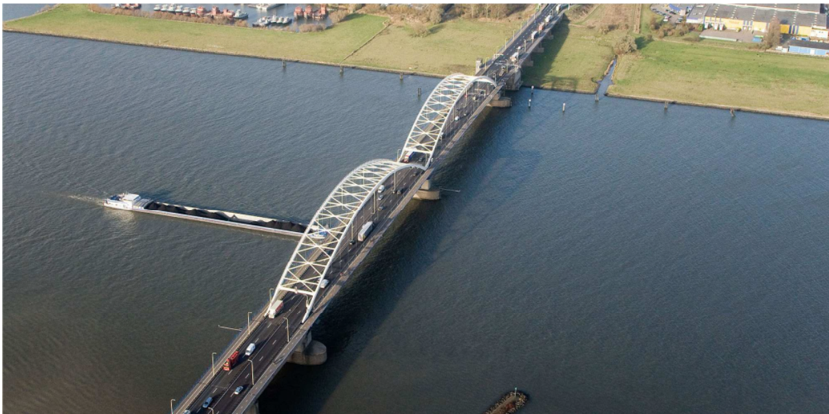
Figure 1. Merwede Bridge (source: beeldbank.rws.nl )
