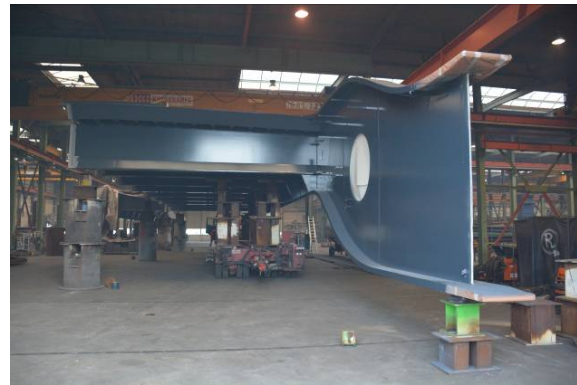
Figure 12. Steel deck after coating
